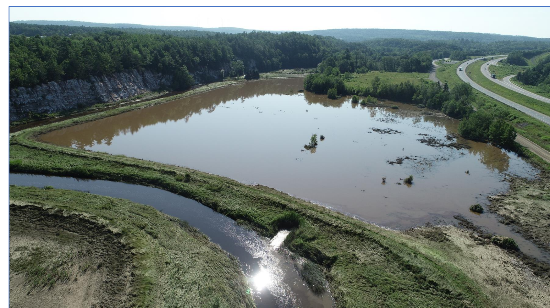
Figure 5: Freshwater flooding in St. Croix dykeland after tragic flooding on July 22, 2023 (photo taken July 23, 2023 by Graeme Matheson, NSDA)
