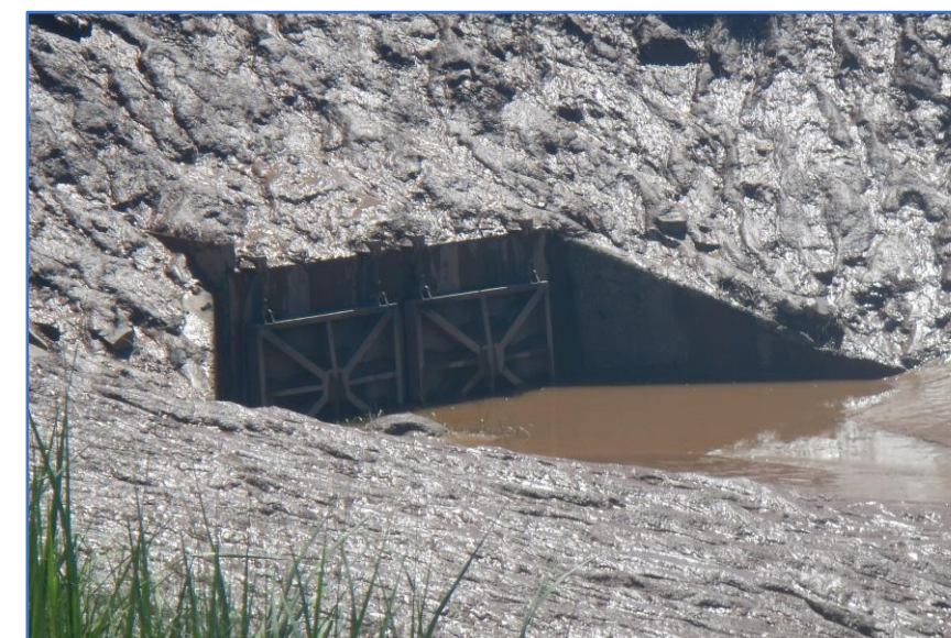
Figure 2: Dykelands drained by aboiteaux – one way gate
