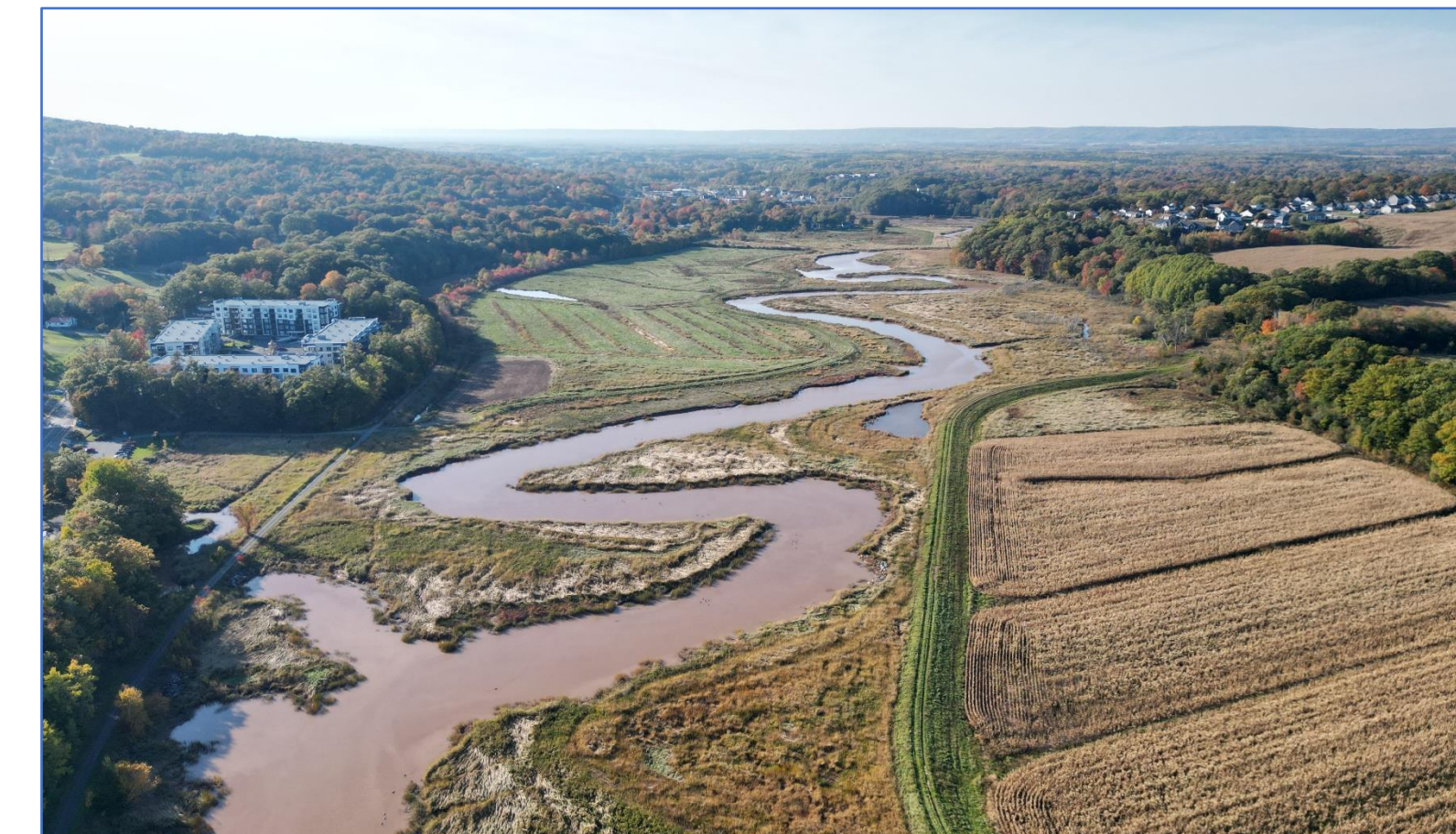
Figure 3: Oblique aerial photo of realigned dyke at Belcher St. Marsh, Cornwallis River in Oct. 2022
