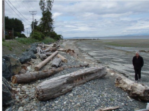
Figure 2.5.2. Large woody material added as part of a soft shore treatment. Credit: H. Rueggeberg.
