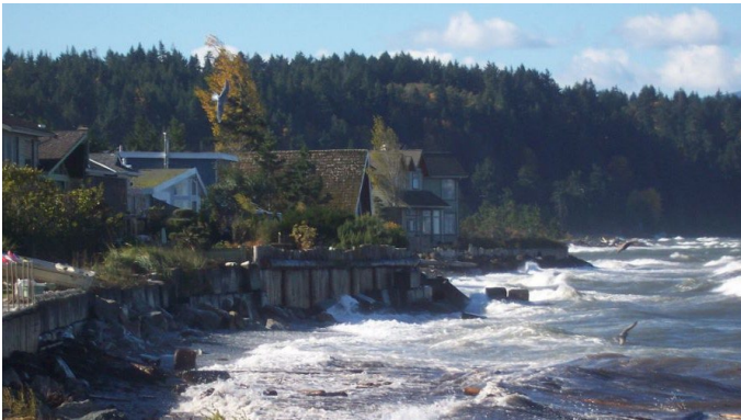
Figure 1.5.4. The suitability of nature-based methods is limited by the amount of wave energy and the proximity of buildings to the shoreline. Credit: Kelly Loch.
