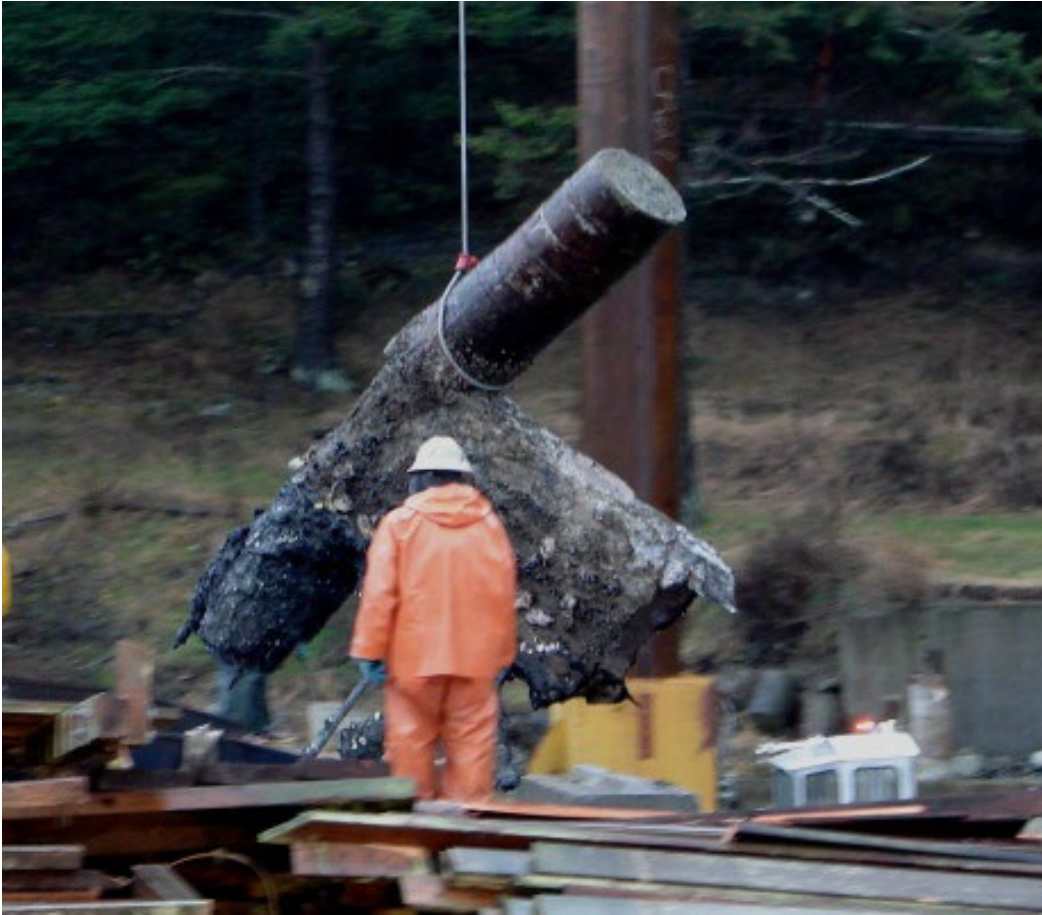
Figure 3.4.1. Removing creosote material. Credit: Washington State Department of Natural Resources.
