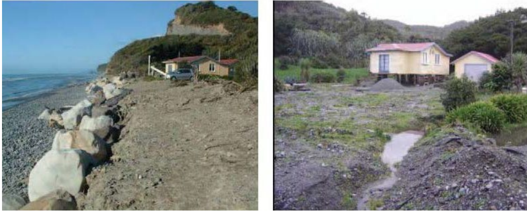
Figure 1.6.1. Relocation of house back from eroding coastline on New Zealand's west coast. Credit: New Zealand Ministry of Environment (2008).
