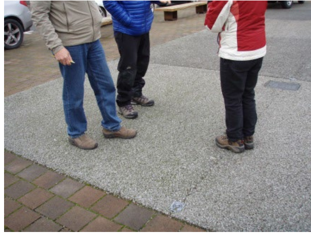
Figure 3.2.3. Pervious parking area. Credit: H. Rueggeberg.
