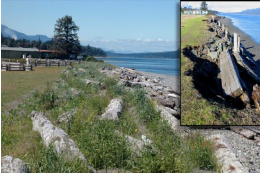
Beach nourishment with logs at Tye Spits in Campbell River, British Columbia Credit: P. Harrison.
