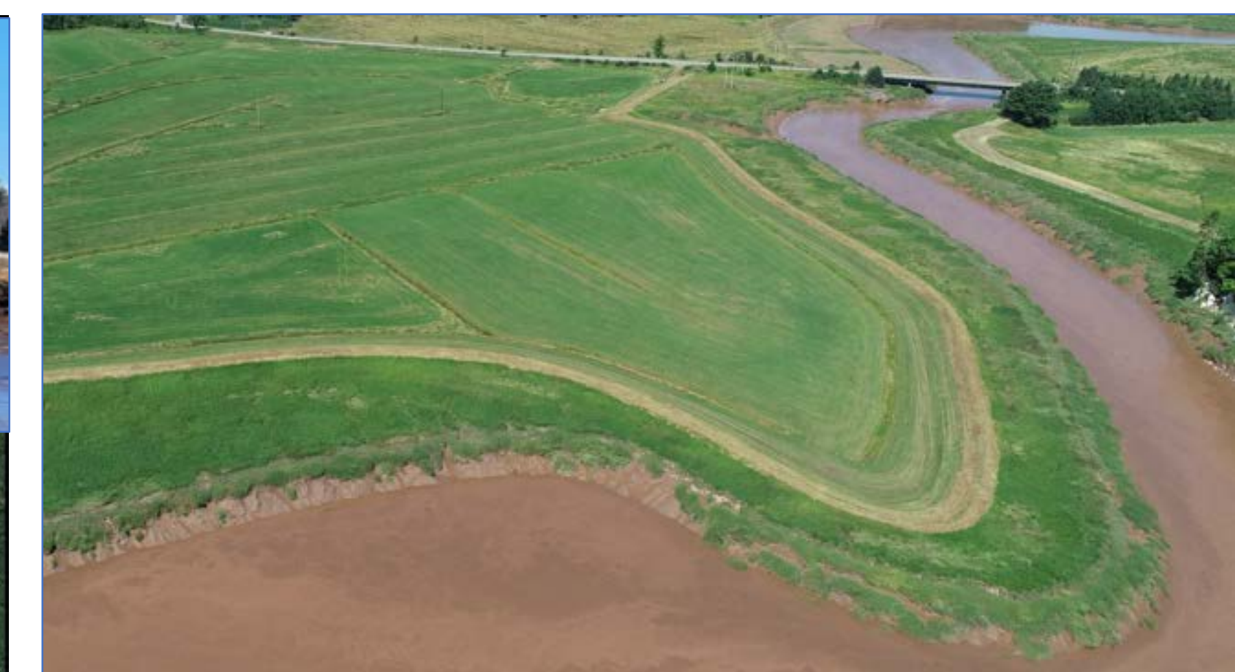
Figure 7: Eroding foreshore marsh and vulnerable dyke section on Tract 4 (photo taken on July 27, 2022 by Graeme Matheson, NSDA).
