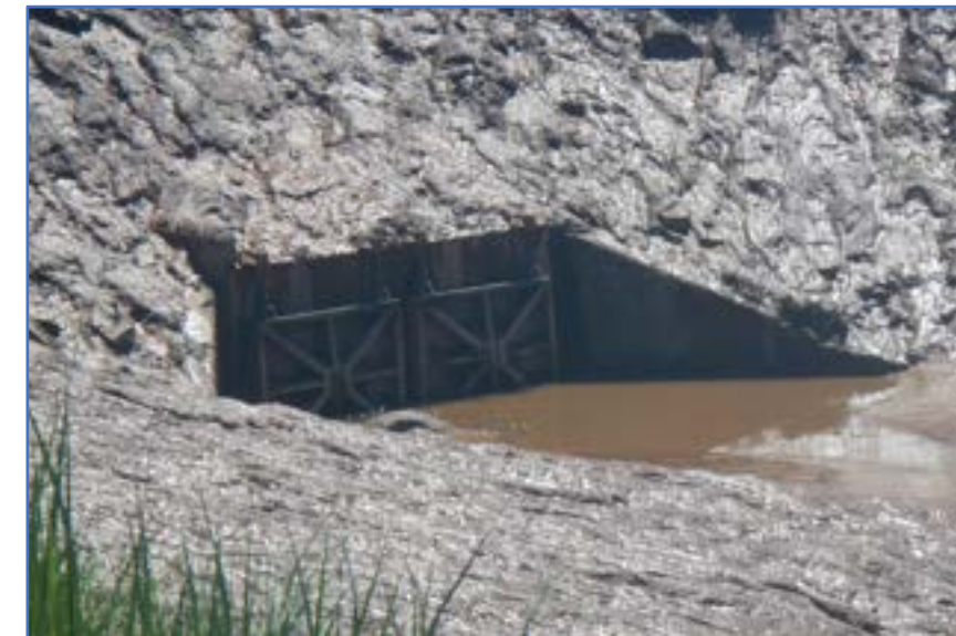
Figure 2: Dykelands drained by aboiteaux – one way gate
