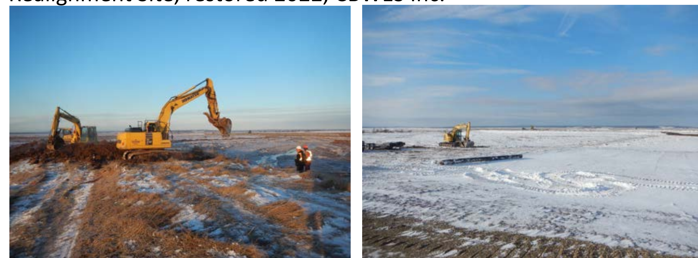
Earthworks at the Converse Marsh Managed Realignment Site, restored 2019, CBWES Inc.
