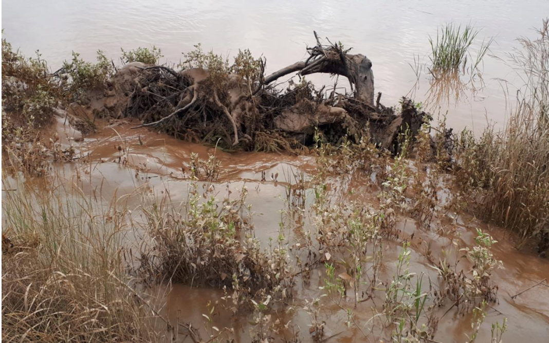
Figure 12: Root wad revetment at Belcher Street Marsh (CBWES & SMU, 2020)
