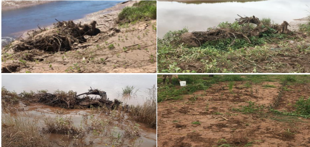
Figure 15: Adaptive management at Belcher Street Marsh managed realignment site – scour around root wads (top left); adaptive management at root wads, 23 July 2019 (top right); sediment deposition behind root wads, 8 August 2019 (bottom left); adaptive management with wattle fences, transplants, and brush matting (bottom right). (Graham et al., 2020)
