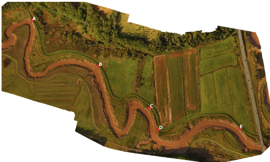
Figure 2. Jijuktu’kwejk River meanders encroaching on the dyke before 2018 and dyke realignment. Points A to E are areas of concern for dyke erosion (Graham et al. , n.d.)
