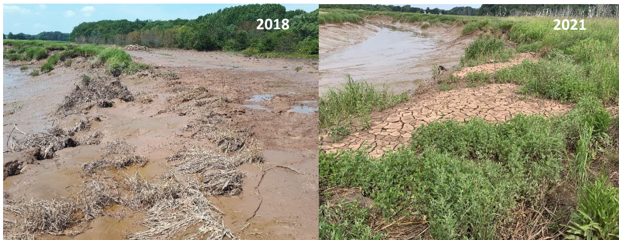
Figure 13. Root wad revetment immediately post-construction in 2018 and year 3 post-construction in 2021
